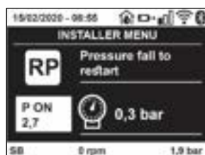
Figure 18 Setting the restart pressure
